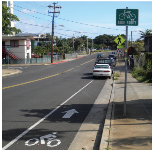
Figure 10.4 - Bike path on Mokuola street blocked by parked cars
