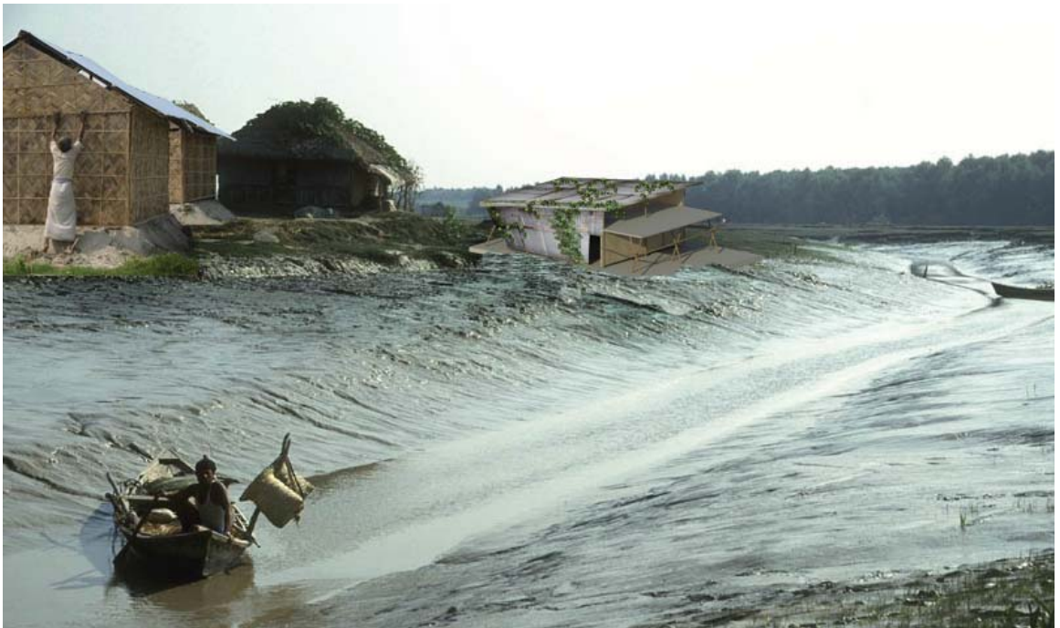
Image 64: 2 prototypes altered, one fitted with corrugated metal and the other altered with mud.
