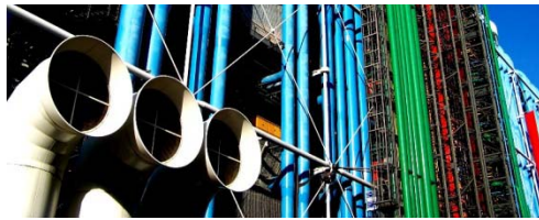
Figure 37. The Pompidou's exposed skeleton of mechanical systems is brightly colored 197
