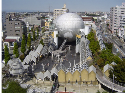
Figure 40. Shonandai Cultural Centre taken from neighboring apartment building 200
