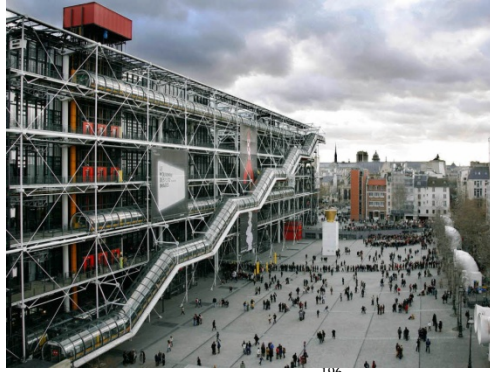
Figure 36. Pompidou Centre, Paris 196
