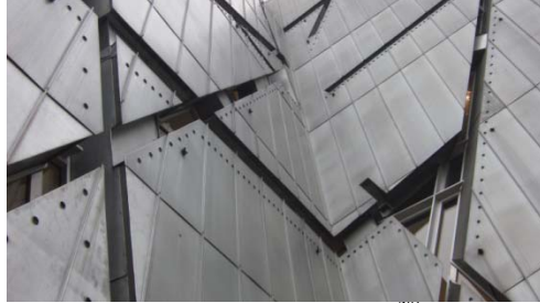
Figure 46. Façade detail of the museum 206
