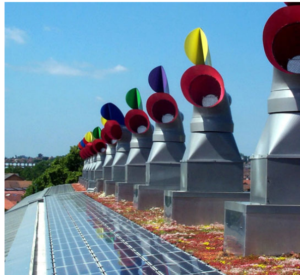
Figure 4.5 - Natural ventilation system
