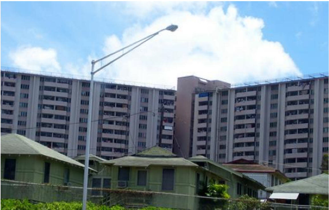
Figure 8. KPT towers and surrounding community. Photo by Governor Neil Abercrombie's office, October 7, 2011. http://www.hawaiireporter.com/over-a-hundred-residents-return-to-renovated-homes-at-state%E2%80%99s-largest-public-housing-project/123 .
