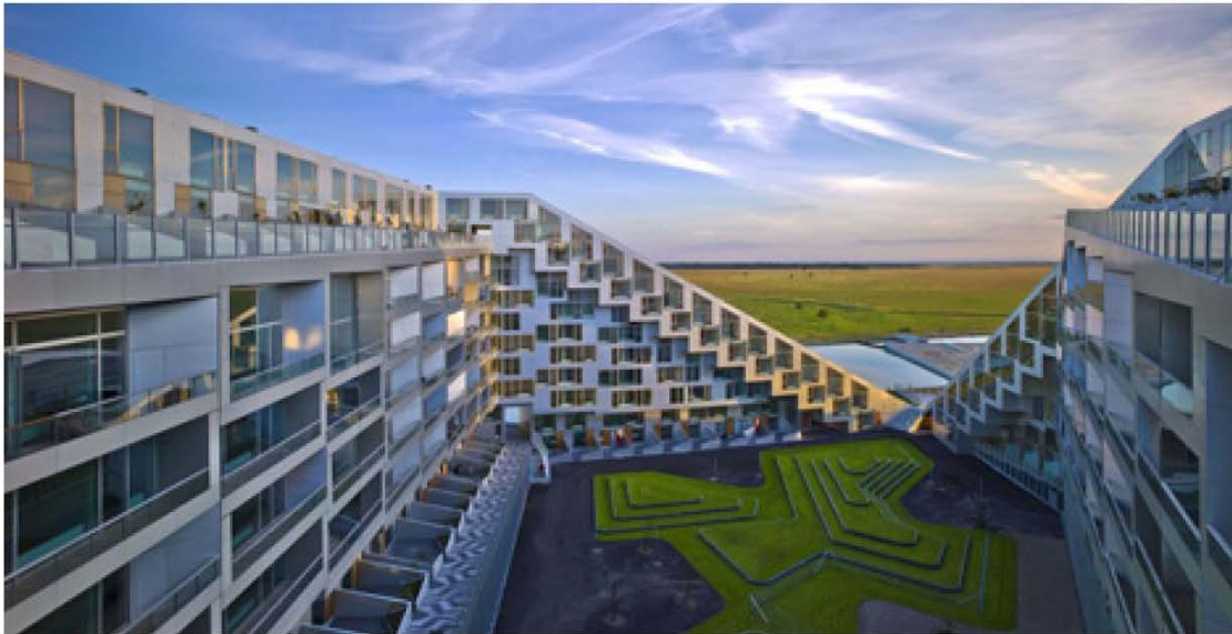
8 House courtyard view http://www.dezeen.com/2010/10/22/8-house-by-big-2/
