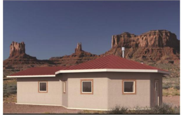
Navajo Elder Housing with straw-bale construction exterior. http://openarchitecturenetwork.org/projects/navajo
