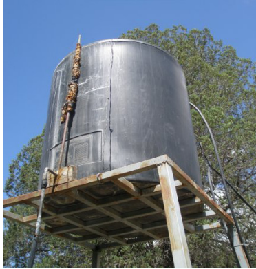
[Figure 5] Community water tank filled with spring water
