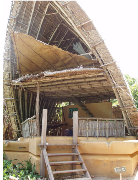
[Figure 33] Operable ventilation
