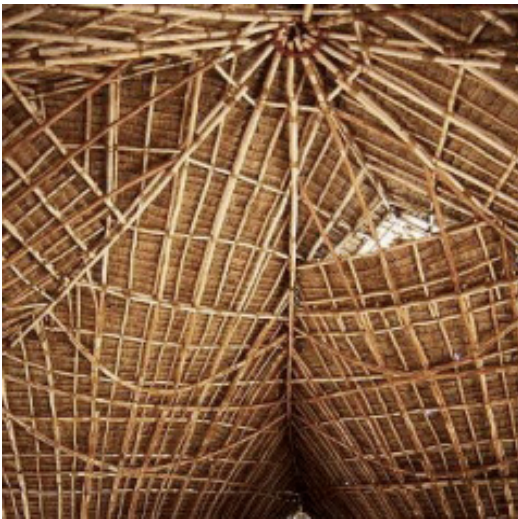
[Figure 35] Roof Structure
