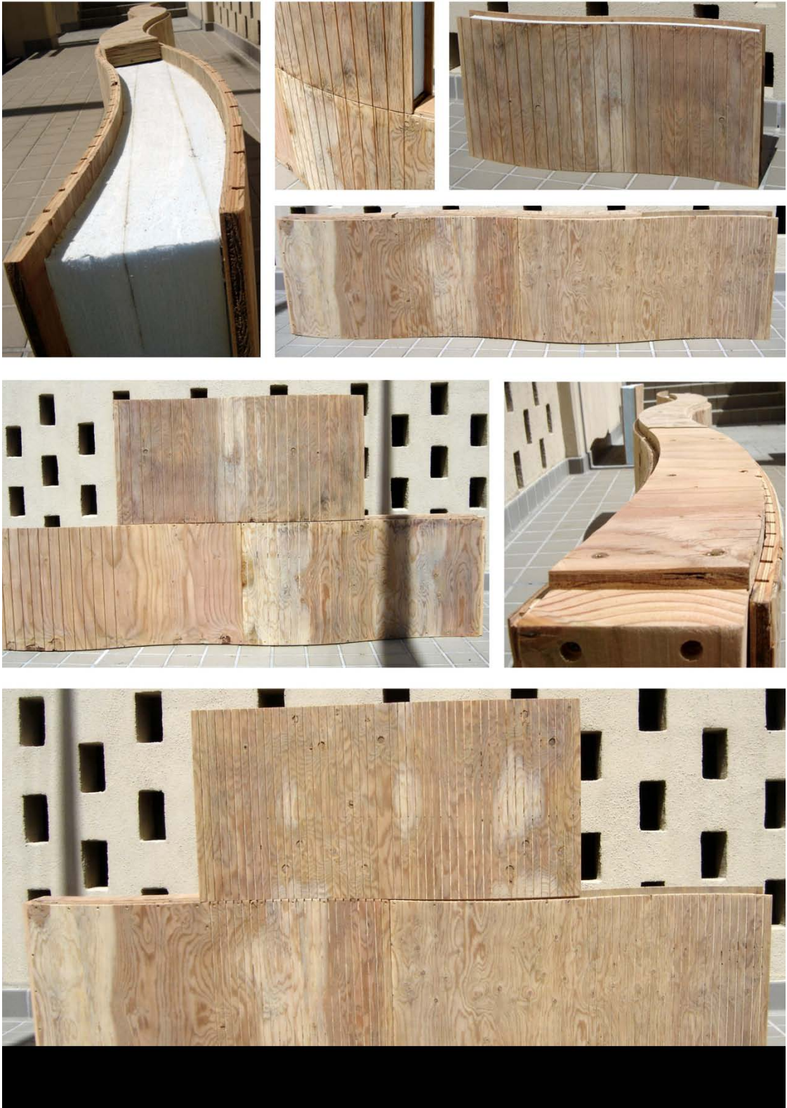
Figure 48 Horizontal SIP wall assembly
