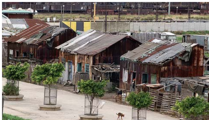
Figure 15. New Brighton, Red Location is composed of a grid of shacks made of thick, aged corrugated iron, rusted red, surrounded by tiny fenced or walled lots.
