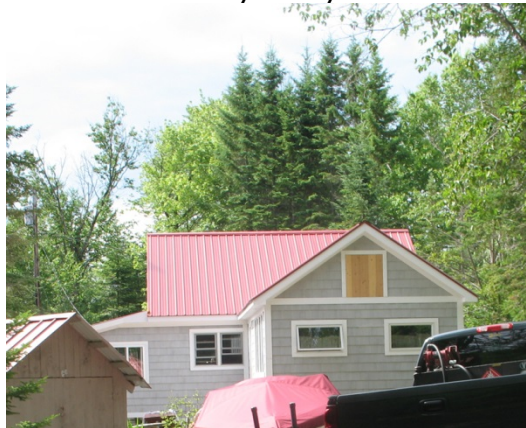
Figure 468. Site Context - view of camp on Onion Point Road taken in July 2012 by author
