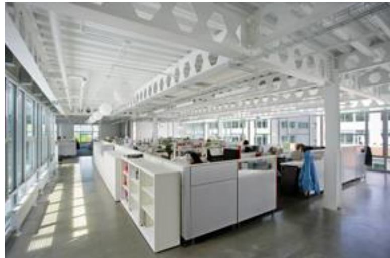
Figure 19. Daylighting strategies taking advantage of natural light by bouncing light into interior and using light colors. Source: NREL
