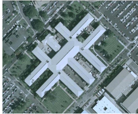
Figure B-7. Overhead view of Pacific Air Forces Headquarter bldg.
