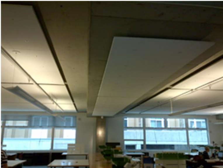
Figure 69. Light colored ceiling panels. Photograph by Travis Watson.
