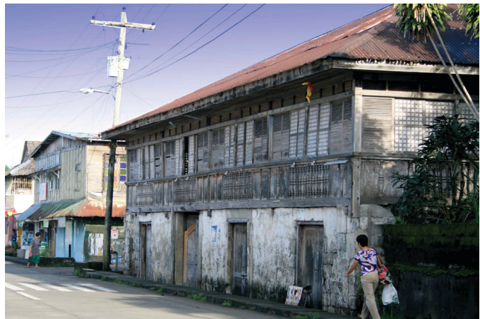
Old Spanish Regime House in Leyte, Philippines. Another version of the bahay na bato in the southern part of the Philippines. The stone lower floor and wooden upper floor remains the same as its northern counterparts.
