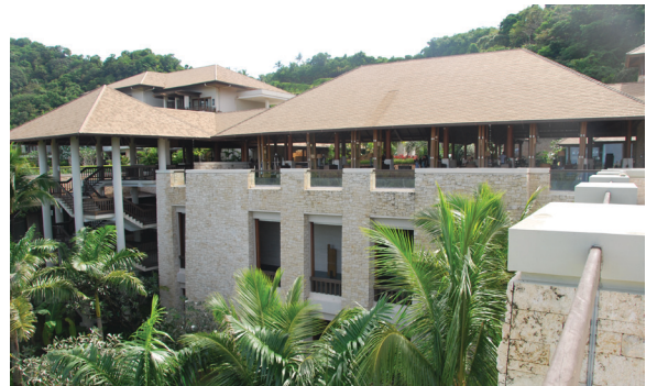
The main lobby area is the center point of the hotel, with "wings" flanking the lobby.
