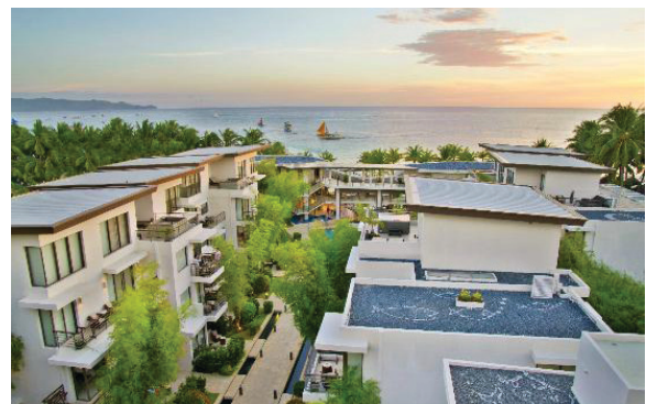
Parallel organization of buildings flanking terrace gardens and walkway towards the pool area.
