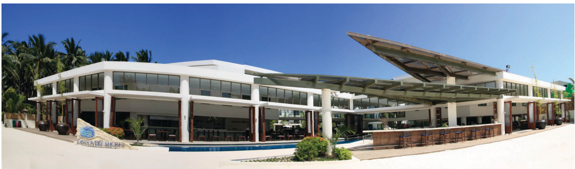
Another view of the lobby and entry area of Discovery Shores
