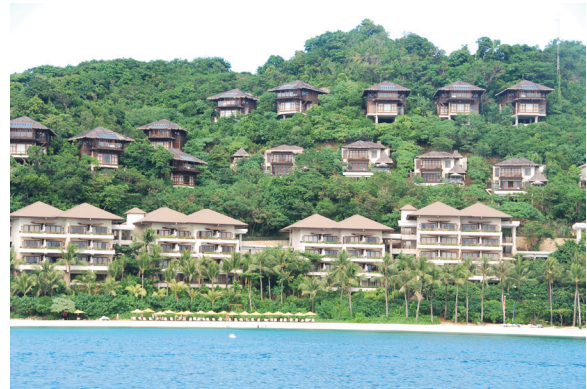
Appropriately situated villas in the hillside, surrounded by the lush tropical environment.
