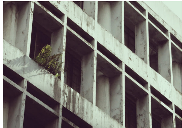
The Madrigal Building, built in the 1950's, exhibits some international and Art Deco style. The brise-soleil , or sun breakers, shown here, prevents overheating.
