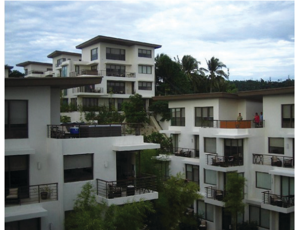
The square, rectangle buildings and flat roofs of Discovery Shores provide a more modern aesthetic, rather than traditional or vernacular appeal.
