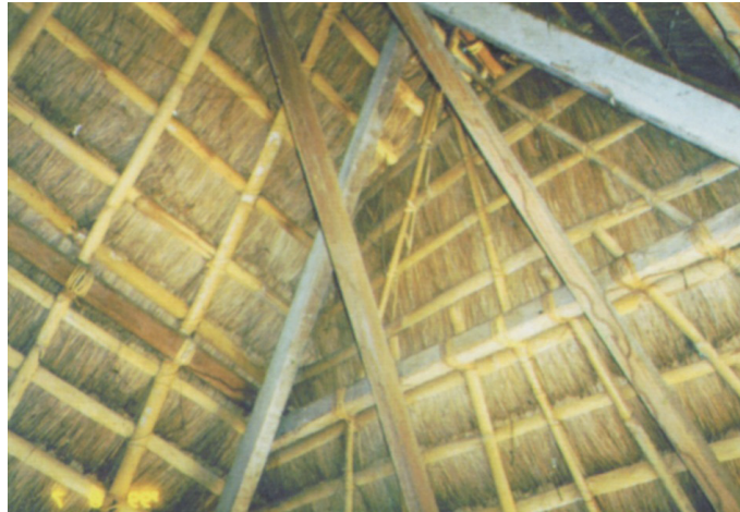
Underside of roof.
