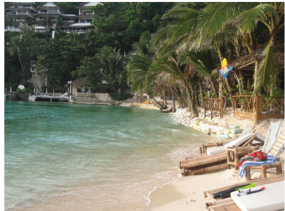
Erosion at Diniwid Beach
