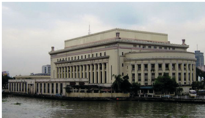
Manila Central Post Office, built during the American colonial period, shows of a neoclassical architectural style.
