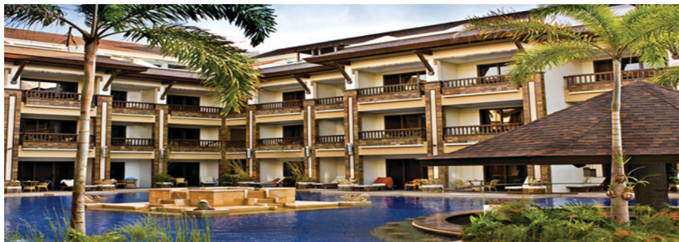
View of main courtyard from corner of lobby
