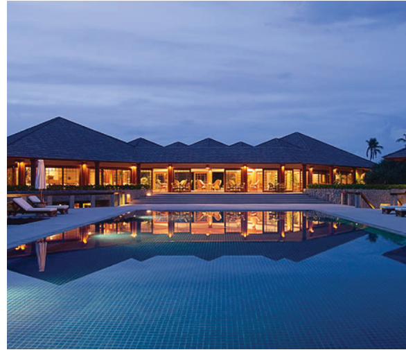
Amanpulo Resort on Palawan. A successful blending of traditional design concept with modern architecture. SOURCE: http://www.amanresorts.com/amanpulo/picturetour.aspx
