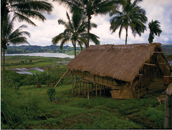
A Tboli bahay kubo, or nipa hut, in Southern Philippines, with a sloped roof and raised floor, made out of the materials found nearby.
