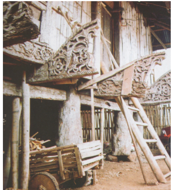
Fancy details with tree trunk posts on top of stones.
