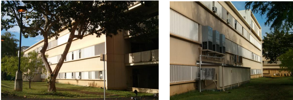
Figure 118: Physical Science Building
