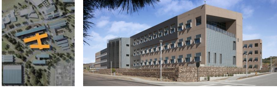
Figure 16: Proper building forms and orientations used in the design of naturally ventilated buildings Source: Research Support Facility (RSF) with narrow layouts and an H-shaped footprint at the National Renewable Energy Laboratory (NREL). Source: the US. Department of Energy.
