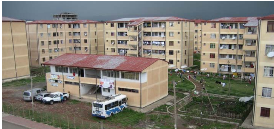
Figure 2.4 decay in newly constructed low-income housing 24
