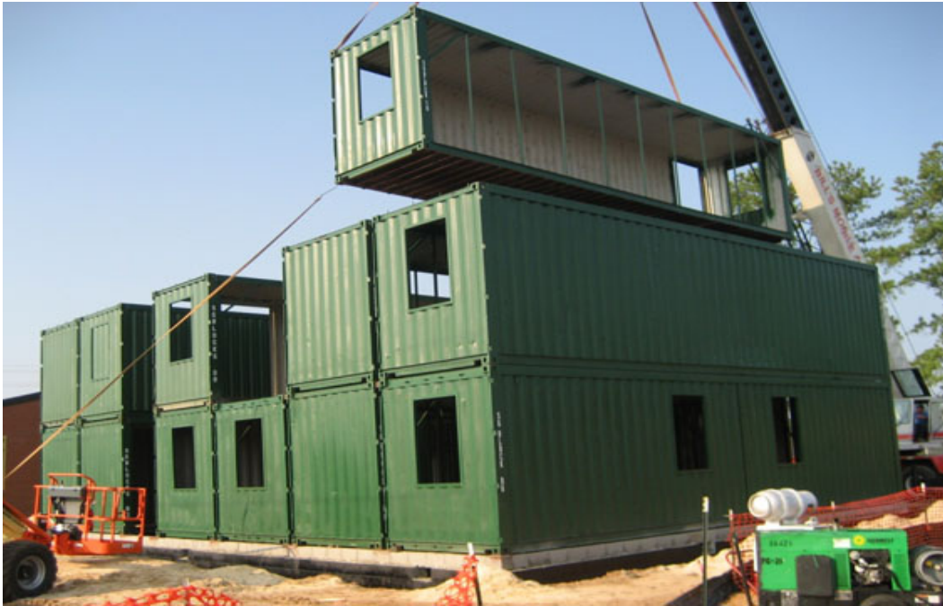
Figure 0.01 Modified containers turned into SGBlocks. http://www.greenhomebuilding.com/articles/containers.htm
