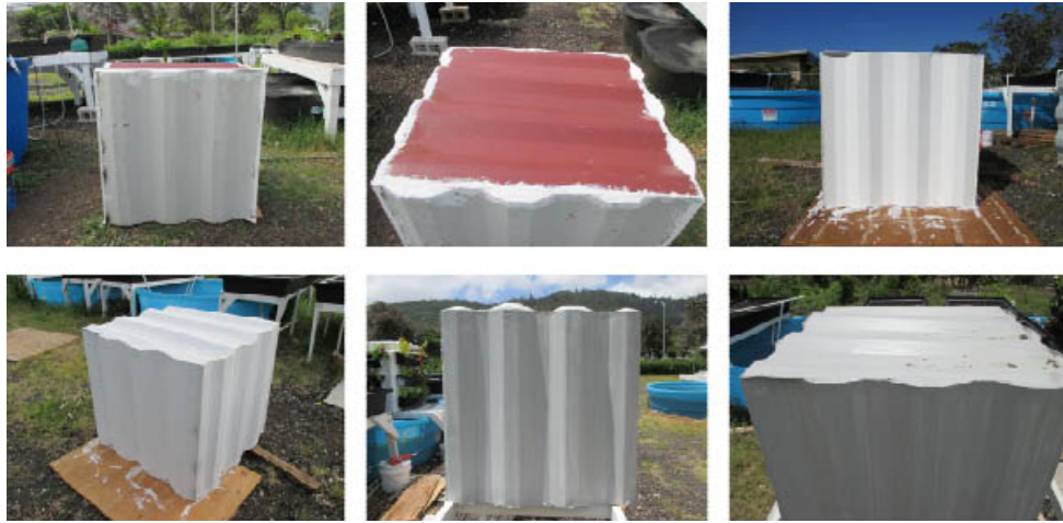
Figure 7.14–Apply patching compound, primer and elastomeric paint. Photograph by Richard E. Mead III
