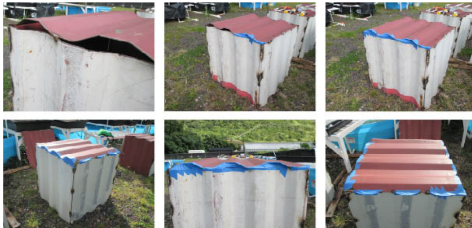
Figure 7.06- Process of sealing container boxes. Taping voids. Photographs by Richard E. Mead III
