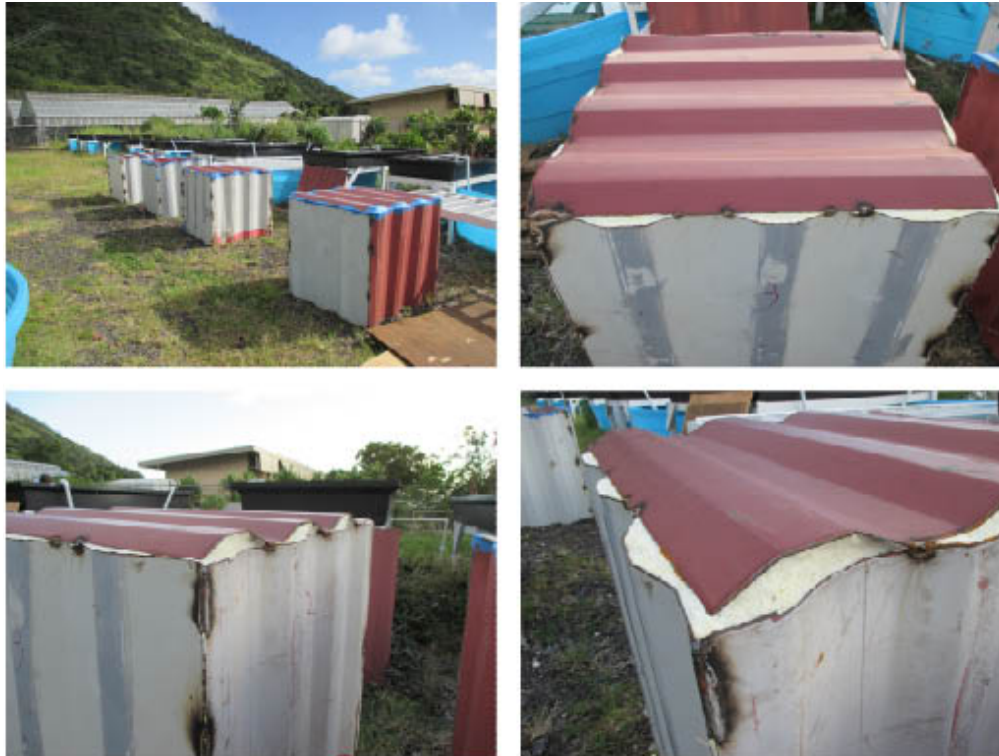
Figure 7.08- Result of spray foam. Smooth finish with all the voids sealed properly. Photographs by Richard E. Mead III
