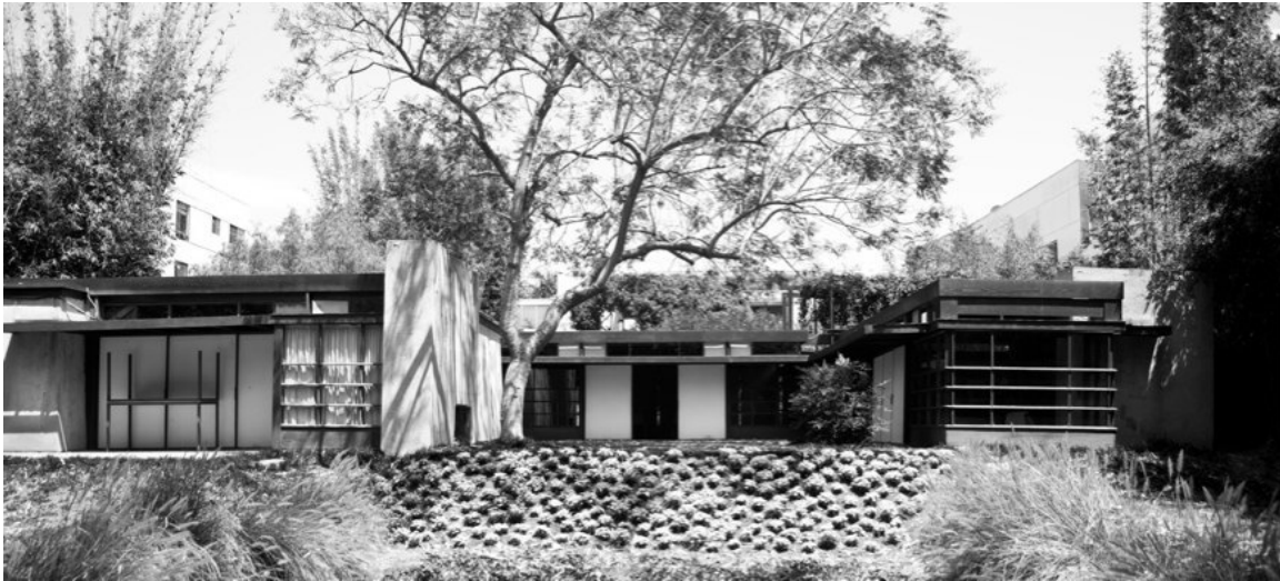
Figure 11 The Schindler House, exterior. (Image from: "Photos: Schindler House," Moby, accessed April 7, 2014, http://www.moby.com/photos/2012-05-22/schindler-house.html )
