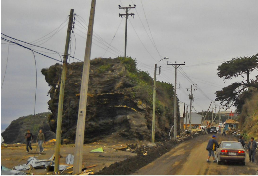
Figure 28: Electric infrastructure affected by 27F Tsunami. Source: Felipe Iguait 2010.
