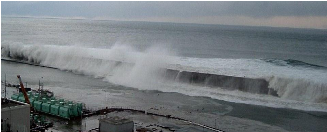
Figure 61: Seawall Collapse in Fukushima Source: DailyMail 103
