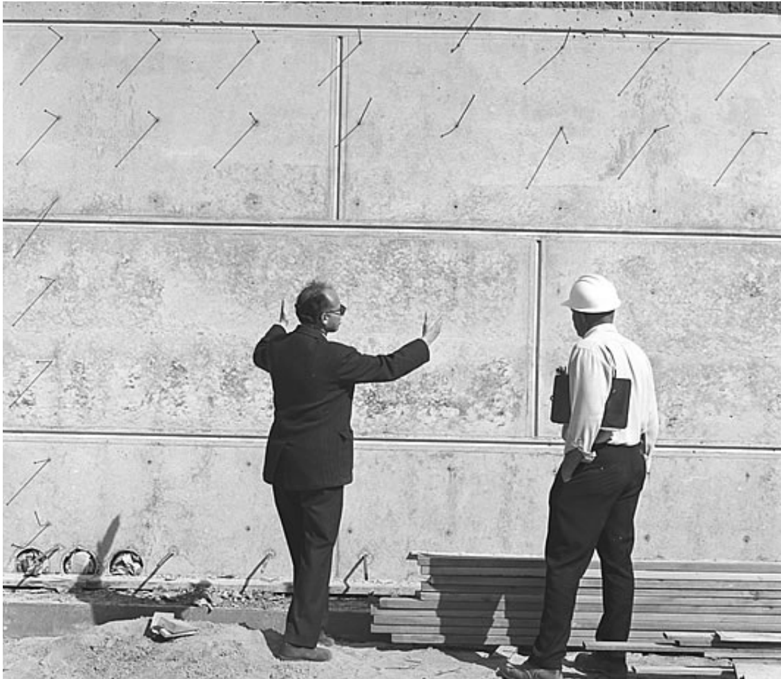
Figure 25 Salk Institute Construction [Photo from History of Salk, http://www.salk.edu/about/history.html ]
