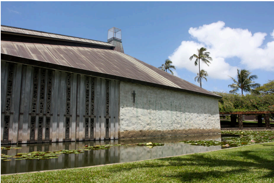
Figure 23 Thurston Chapel Exterior
