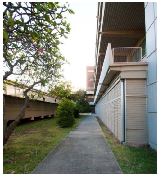
Figure 29: View of Type 1B from main pathway
