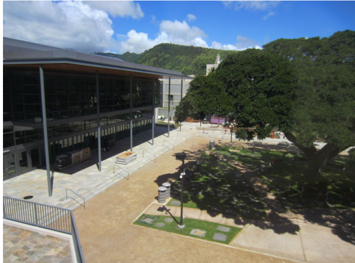
Figure 34: View of Type 3A courtyard
