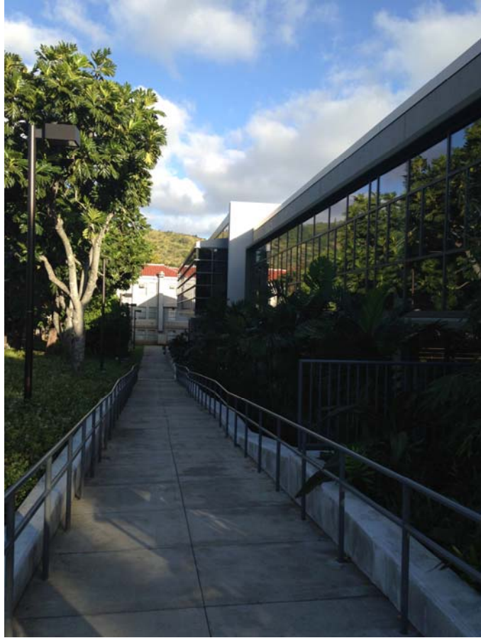
Figure 39: View A. WRC North façade curtain wall overlooking ramp
