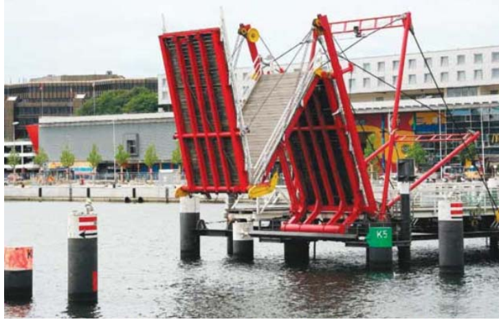
Folding bridge near Kiel, Germany. Engineer: Jörg Schlaich. Courtesy of M. Winzenburg.
