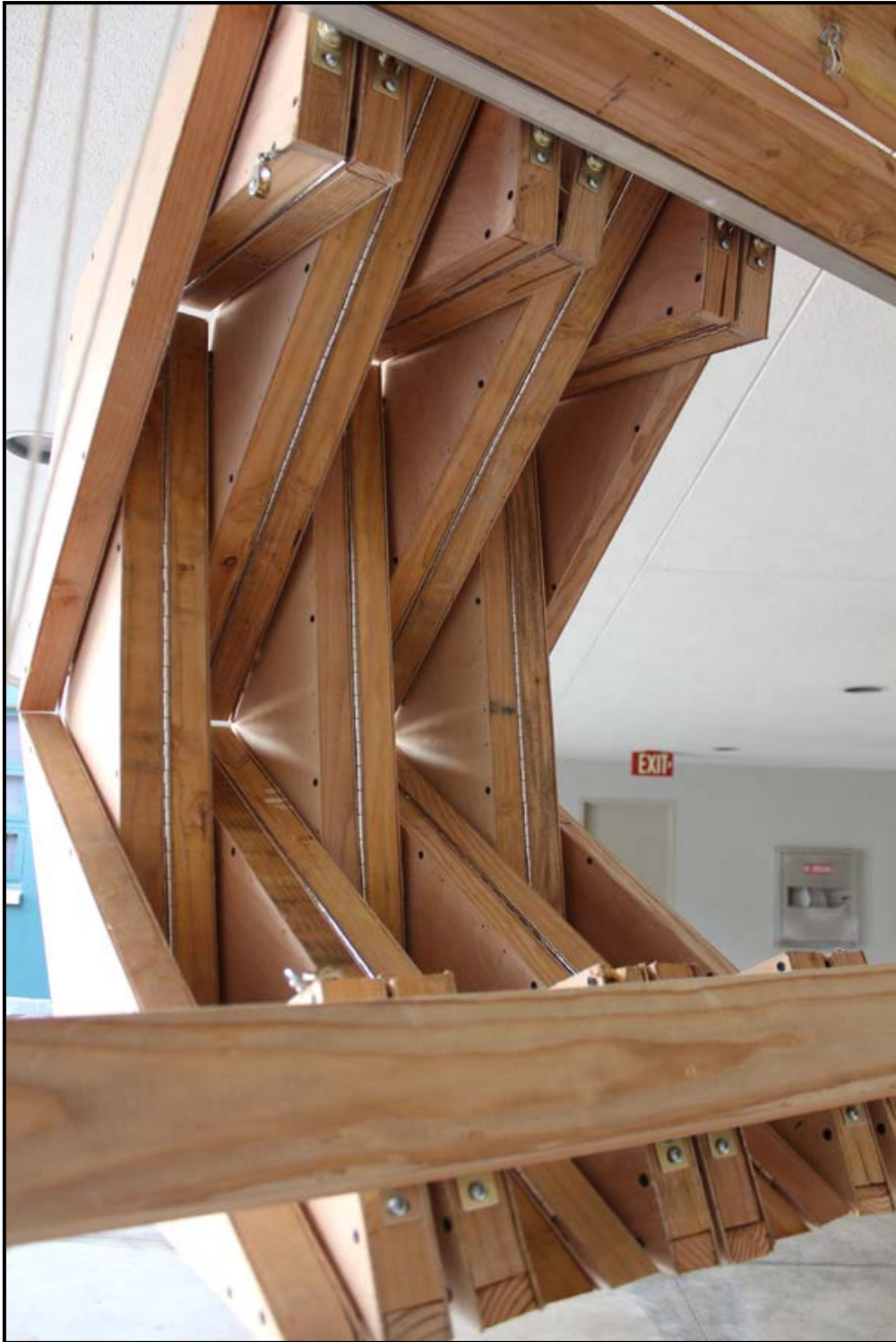
Figure 12.3.6 Close up of reverse side of the large scale prototype in the closed position
