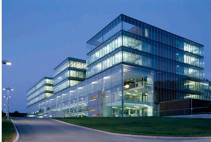
Figure 14: Front Façade of the courthouse. R. Himmelfreundpointer, P. Ott, H. Miltner, Leoben Center of Justice, (Germany, 2006)
