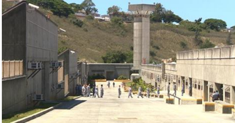
Figure 10: A view from inside Halawas walls."Halawa prison safety fixes to cost $261K," Hawaii News Now, Accessed May 4 th , 2015, http://www.hawaiinewsnow.com/story/27181294/halawa-prison-safety-fixes-to-cost-261k
