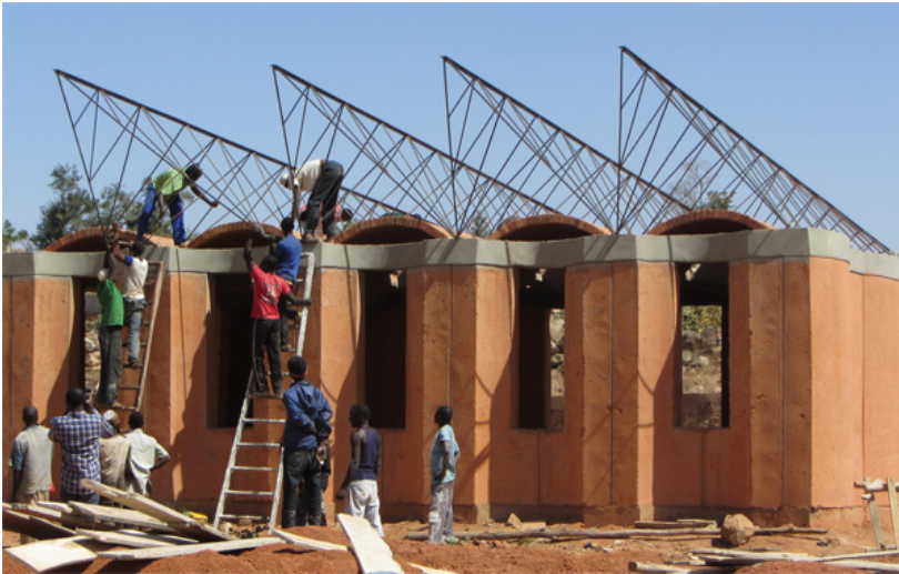
Figure 47: Construction of the school.
