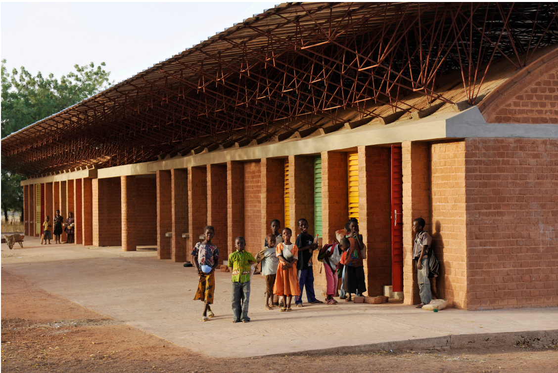
Figure 46: Double roof systems
