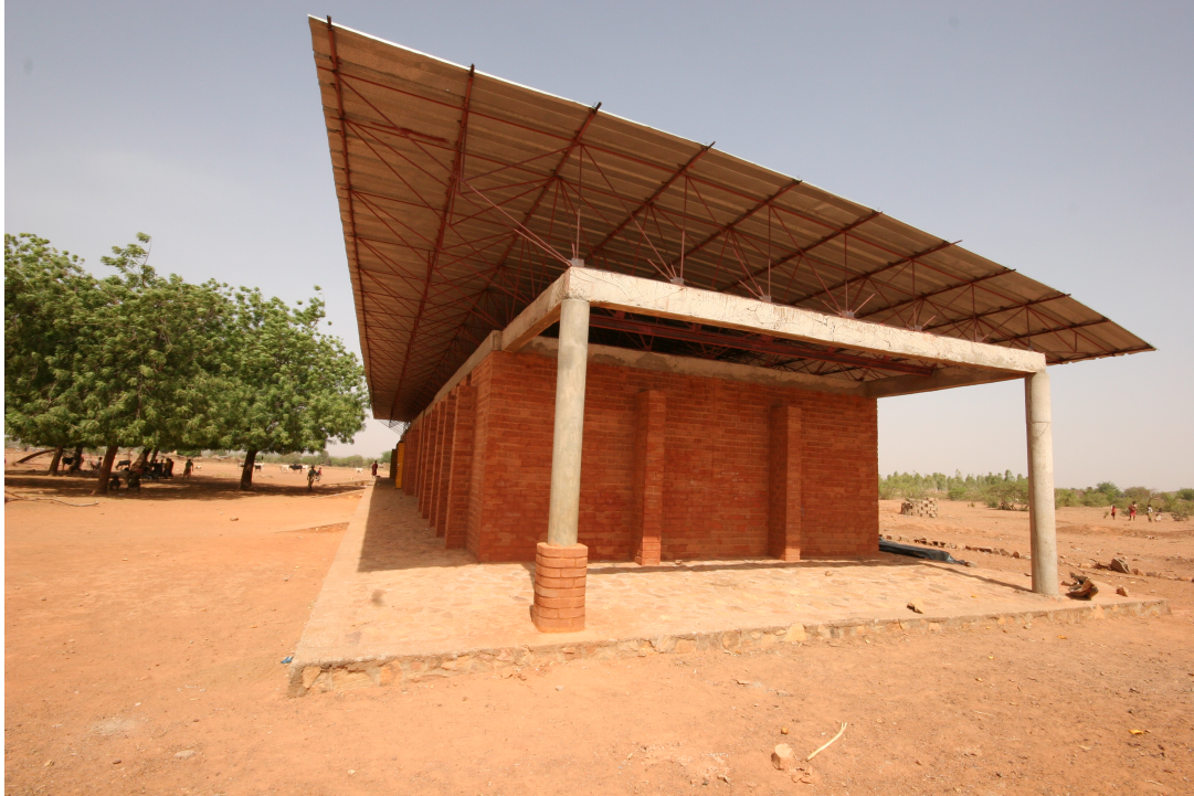
Figure 48: Large Corrugated tin roof for shading.
