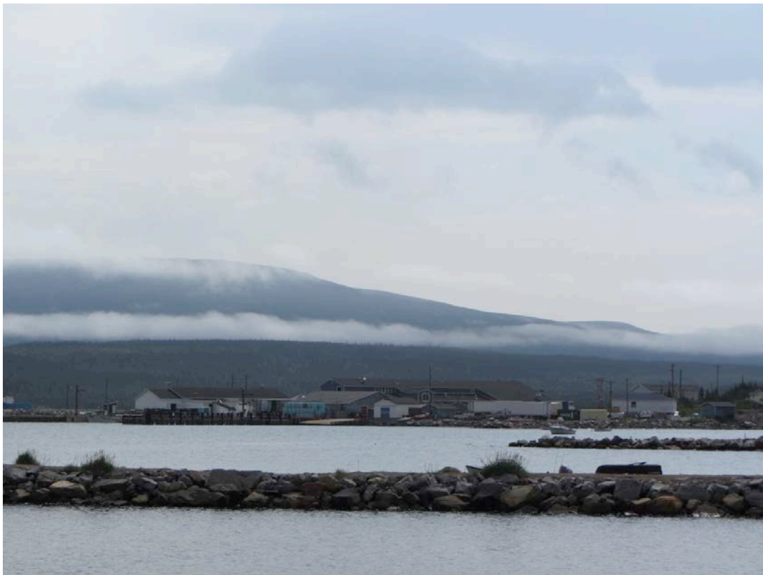
Makkovik Harbour with wharf and fish processing plant infrastructure in the background, August 2015 Photo: Paul Foley
