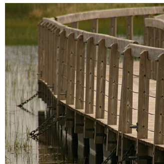
Figure 4.39 Wood Deck & Boardwalk
