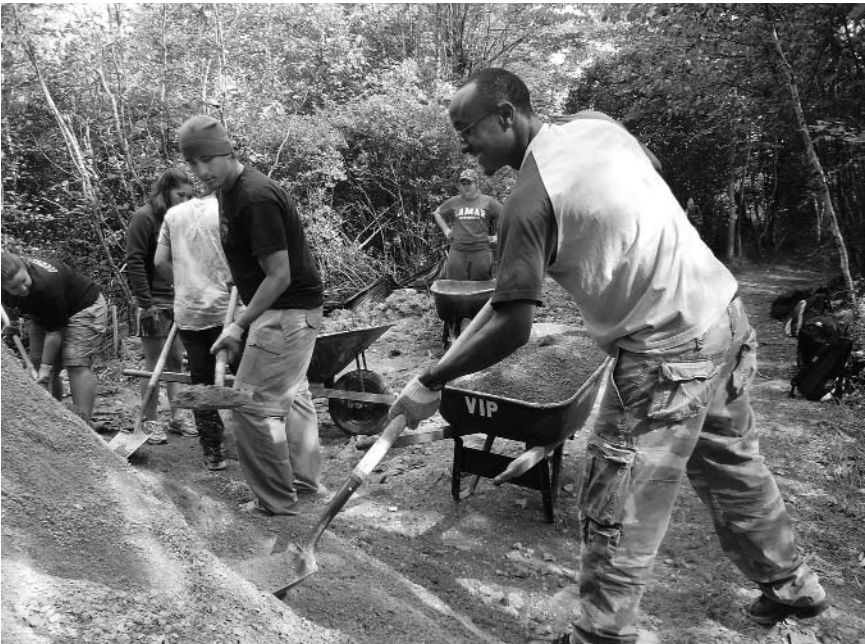
Building a trail, Acadia
