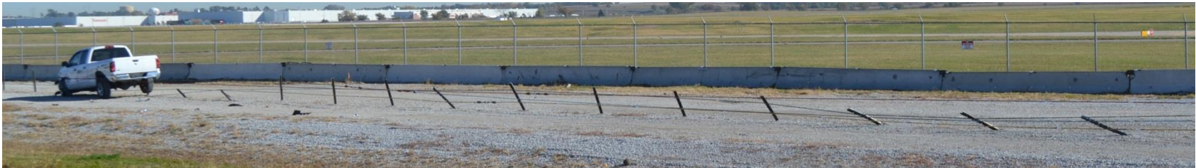
Figure 49. System Damage, Test No. MWP-4
