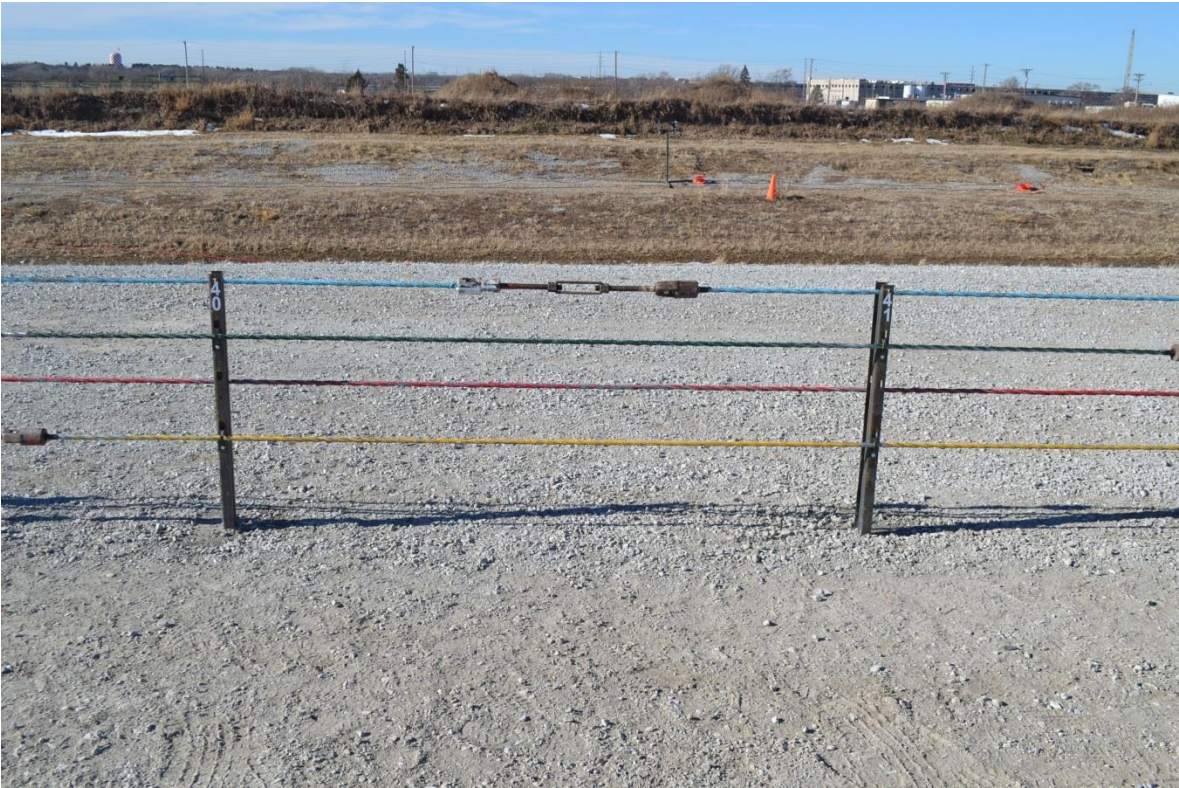
Figure 86. Test Installation Photographs, Test No. MWP-6
