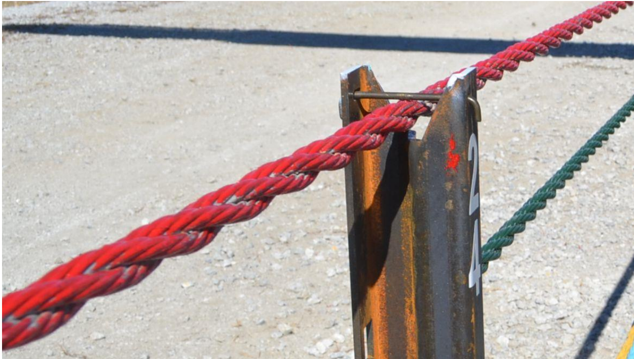
Figure 39. Test Installation Photographs, Test No. MWP-4
