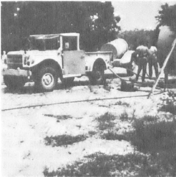
Unloading Sewage Effluent into Storage Tank
