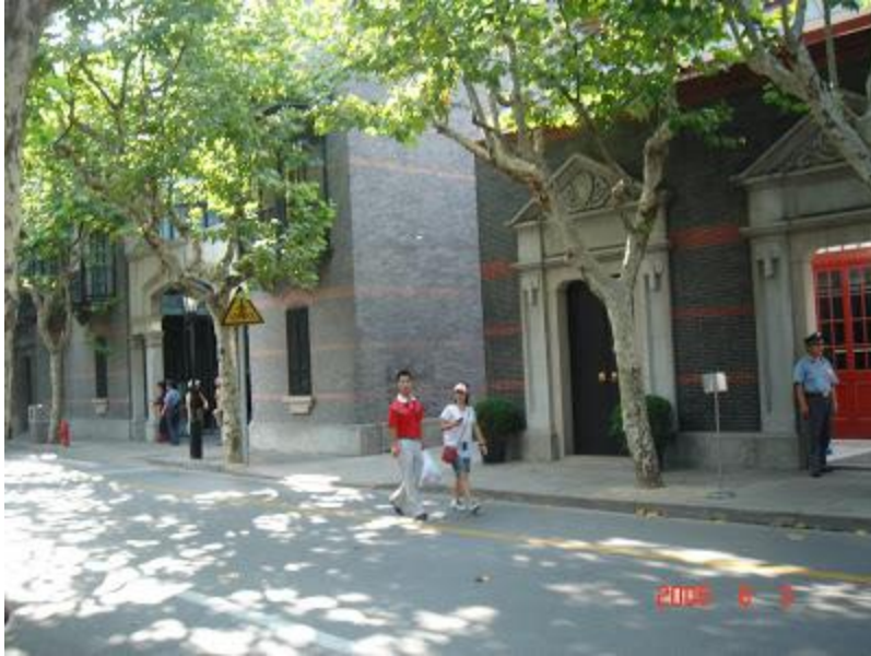
The entrance hall of the new extension of the CCP memorial, 2006 © Samuel Y. Liang
