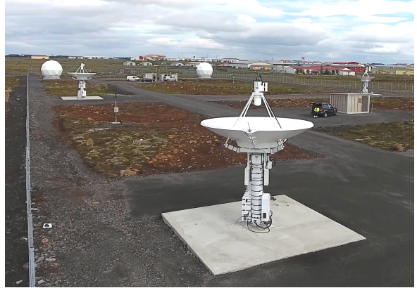
Figure 6: A 4.5 m diameter ground station antenna at Keflavik, Iceland.
