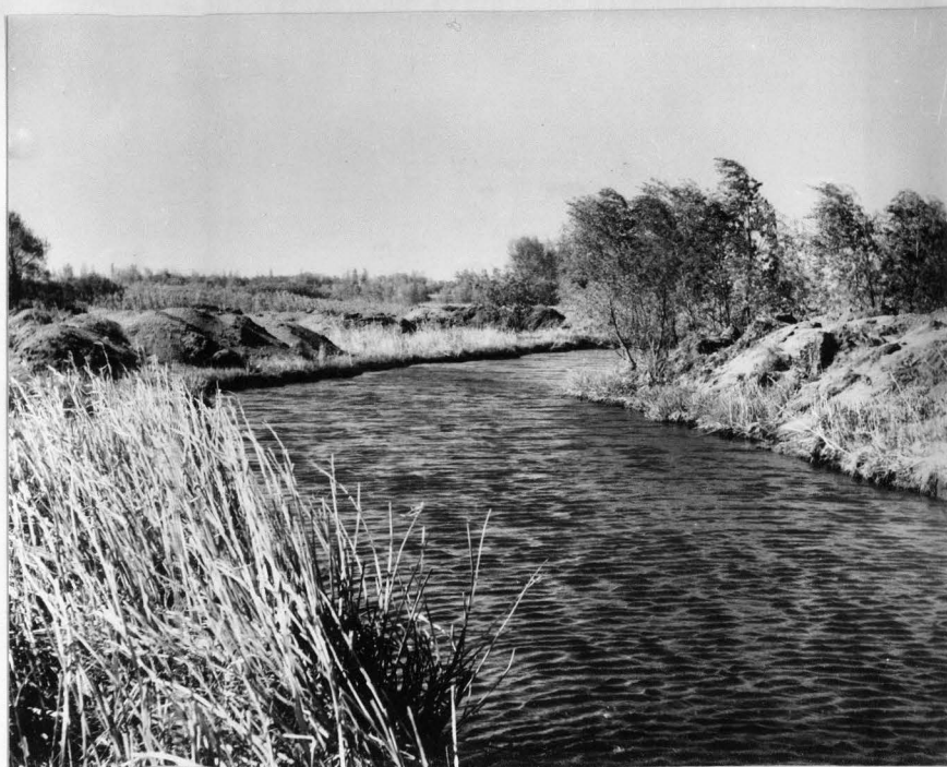
Figure 16. Level ditch about 10 months after construction. May 26, 1957
