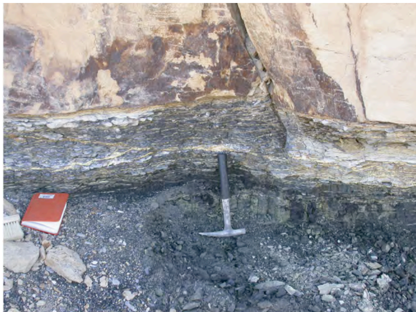
Sandstone joint termination at carbonaceous shale layer in the Ferron M-coal zone at Site 2., Walker Flats Mine.
