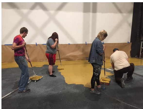
Fig. 3.23 - Beginning Floor Treatment
