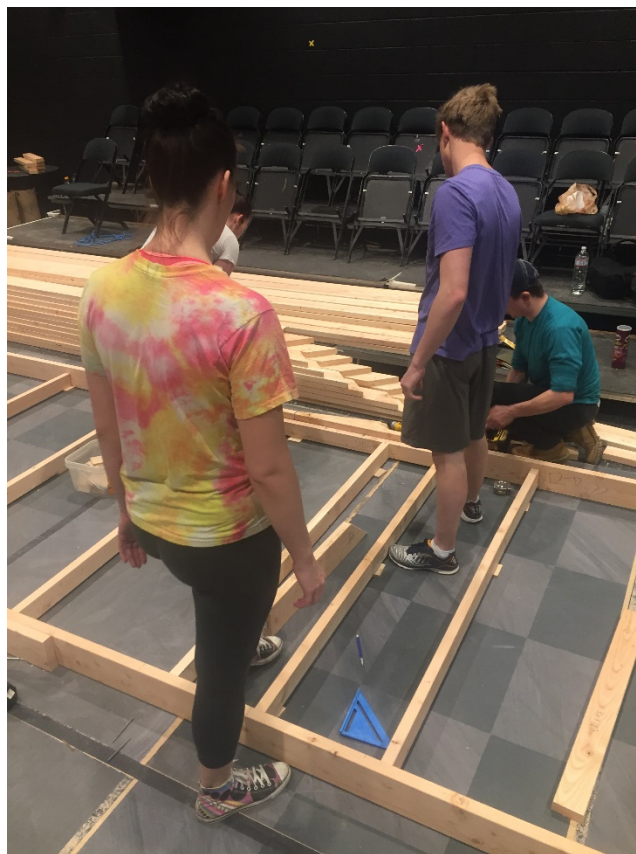
Fig. 2.15 - Framing Upper Deck
