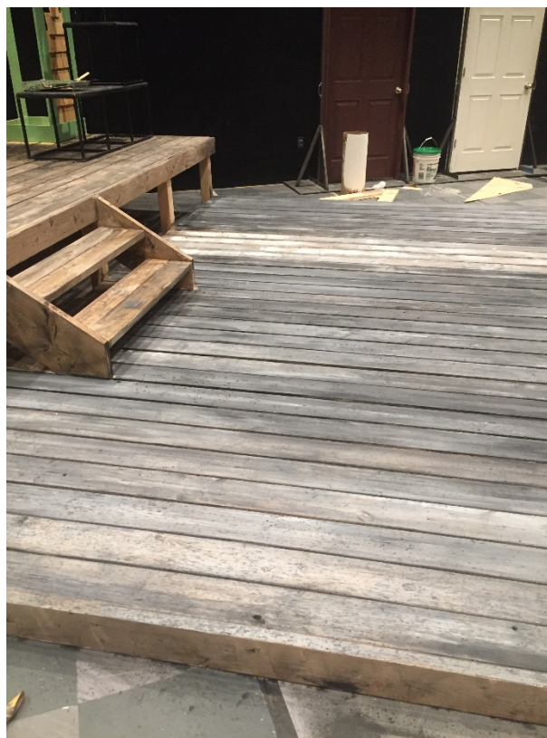
Fig. 2.19 - Deck Painting Process
