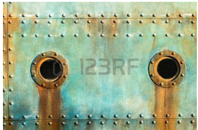
Fig. 1.8 - Rust and Rivet Research (Old)
