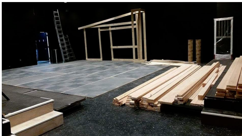
Fig. 2.14 – Boards cut with floor laid out
