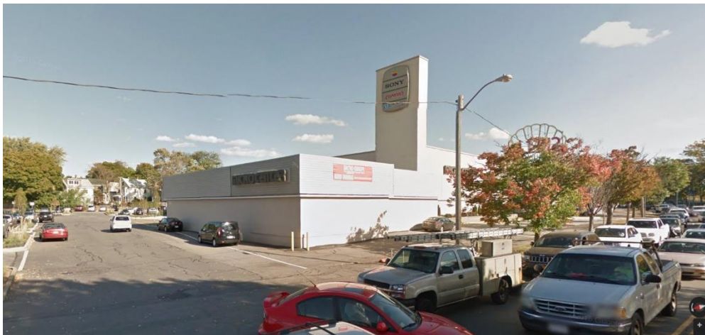
Figure 57. View from the Street (Image credit by author)
