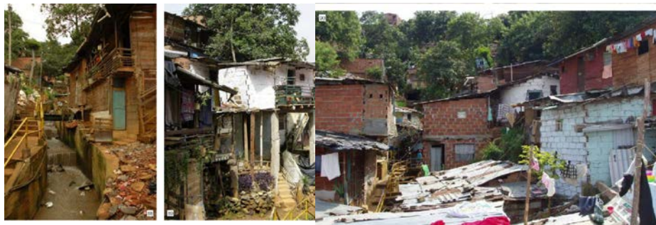
Figure 27: Conditions before PUI project upgrades
