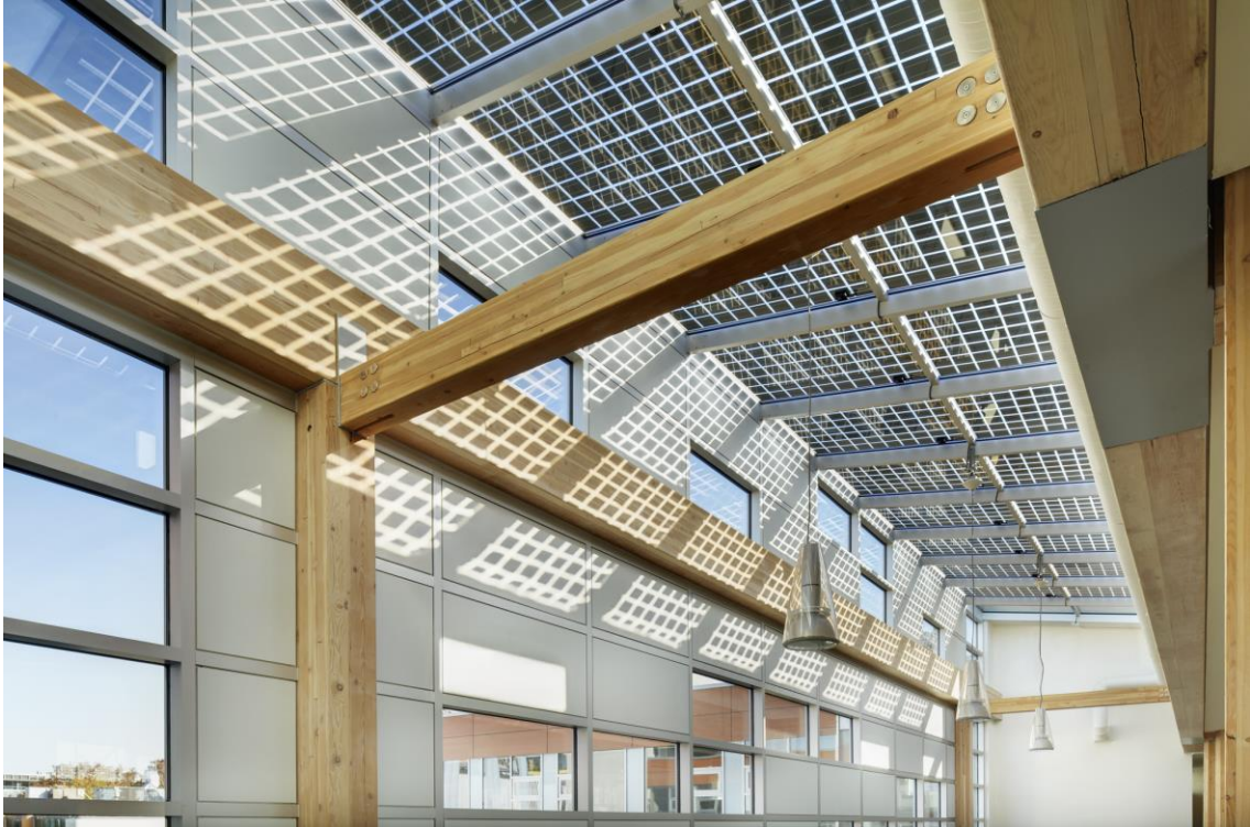
Figure 217, Photovoltaic cells integrated into skylights provide an attractive, yet functional system. Martin Tessler
