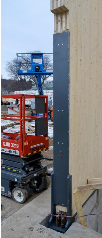
Figure 4: Steel plate bolted to concrete. Alex Schreyer
