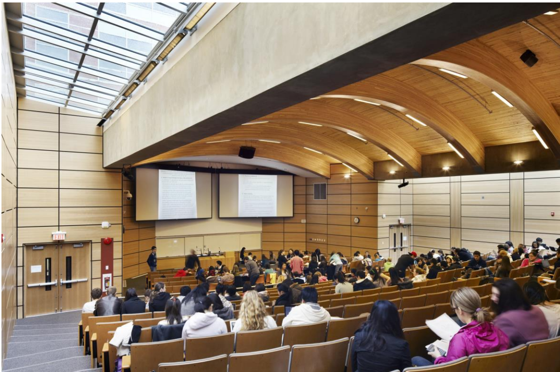
Figure 218, The day-lit auditorium uses glulam arches as an alternate to steel beams or trusses. Martin Tessler
