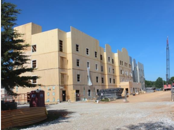
Figure 191, Exposed CLT during Construction.
