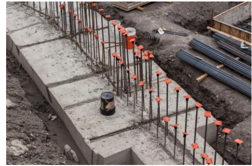
Figure 241, Cast-in-place concrete footing. Dylan Brown
