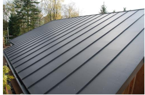
Figure 240, Zinc standing seam roofing.
