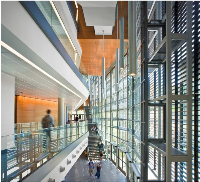
Figure 200, UMass Integrated Sciences Building – Multistory atrium with exposed steel framing. Warren Jagger
