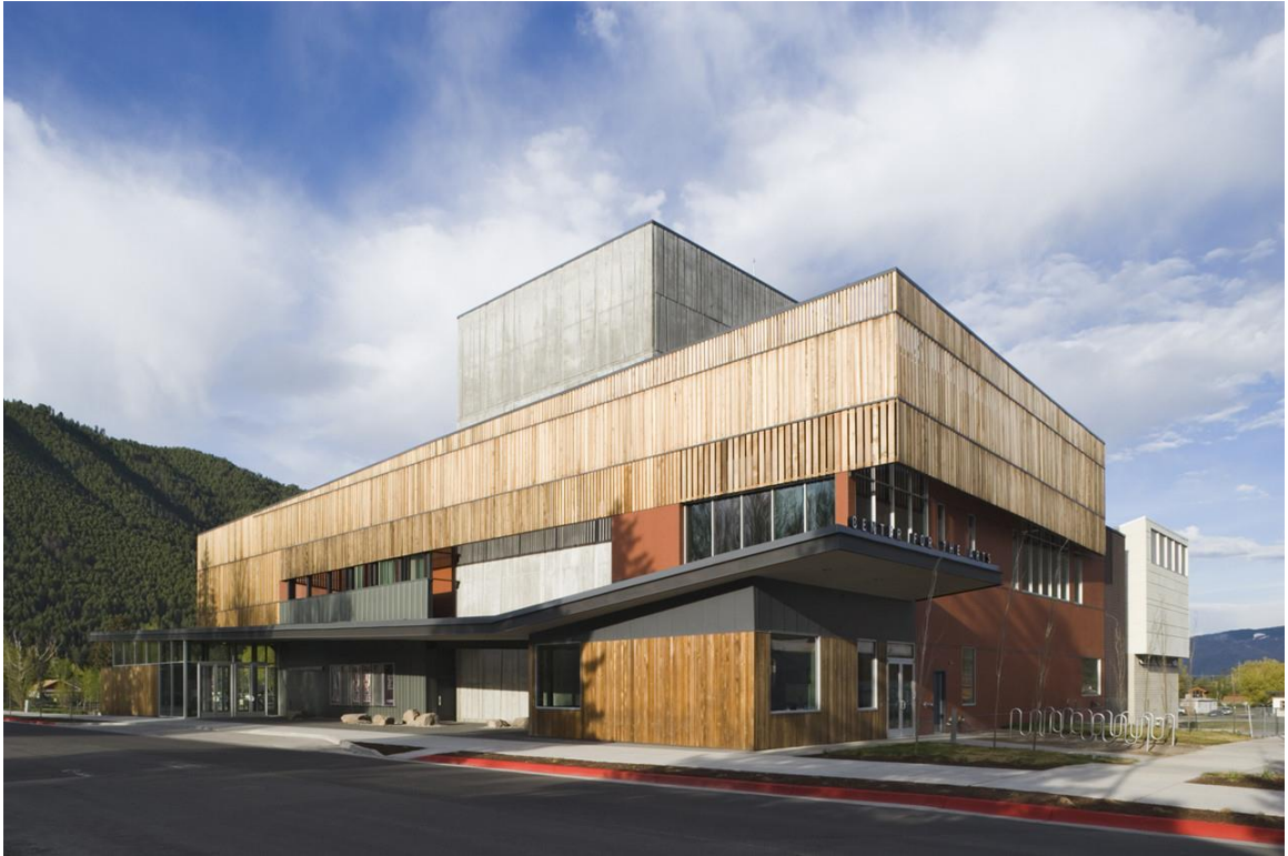
Figure 60, Exposed concrete and wood slat siding reflect the natural setting of the center. Ron Johnson
