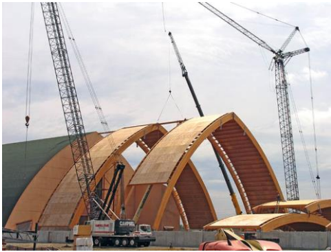
Figure 189, Three hinge glulam arch. Western Wood Structures
