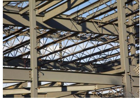
Figure 237, Mild steel used for structural members.
