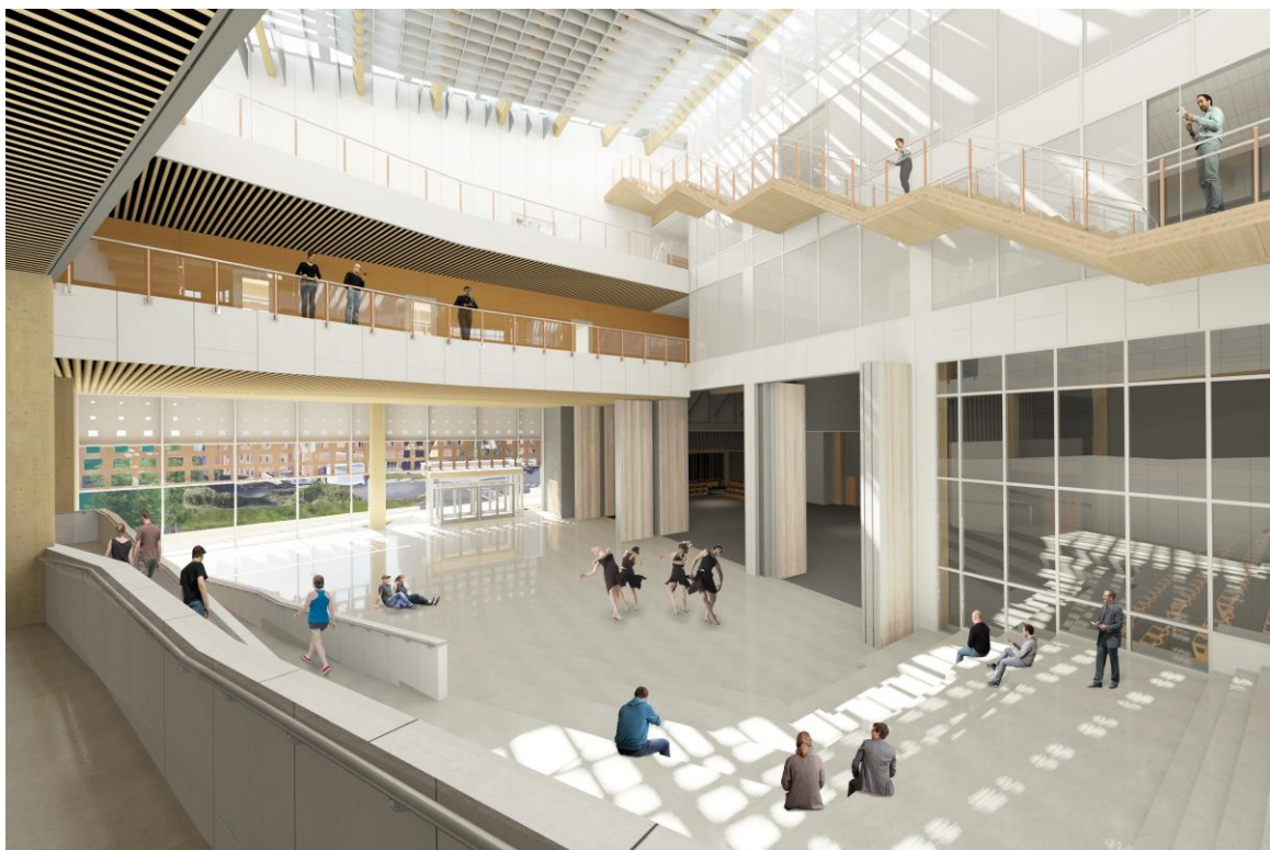
Figure 165, Main atrium as viewed from the second-floor ramp.
