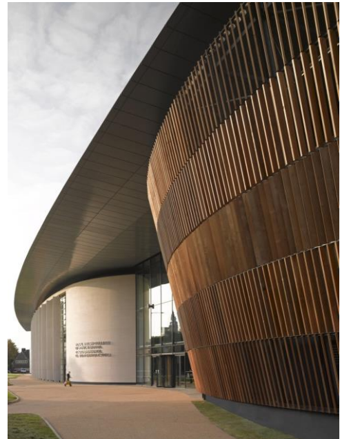
Figure 56, The building facade is a timber screen built from cedar wood slats. BFLS
