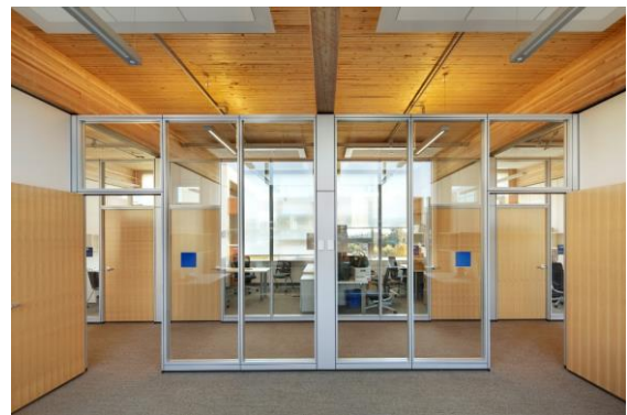
Figure 216, Exposed timber beams and floor panels. Martin Tessler
