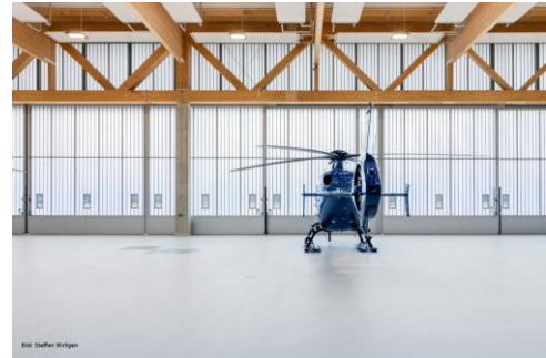
Figure 187, Glulam heavy timber truss. Steffen Wirtgen
