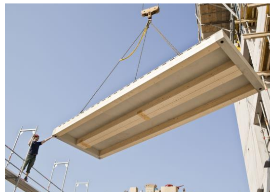
Figure 193, Workers hoisting a prefabricated floor section into place.
