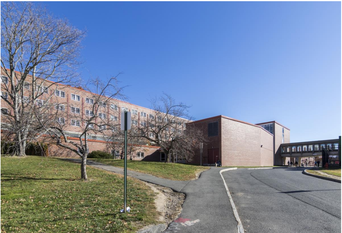
Figure 91, View of Bartlett from the north west. Dylan Brown
