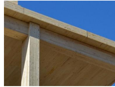
Figure 185, CLT Roof Panel. Alex Schreyer
