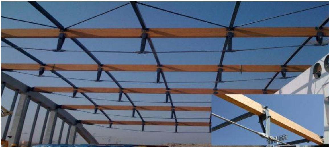
Figure 188, Wood and steel hybrid truss. Structural Timber Solutions LLC
