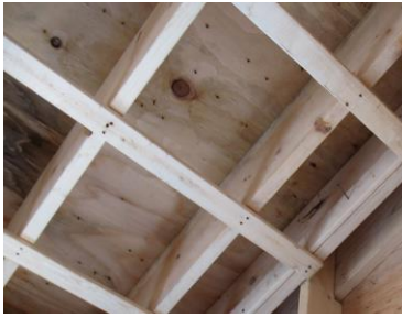
Figure 183, Plywood Sheathing. Dylan Brown
