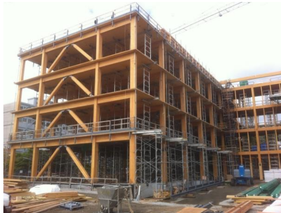
Figure 206, Exposed mass timber structure during construction. Credit
