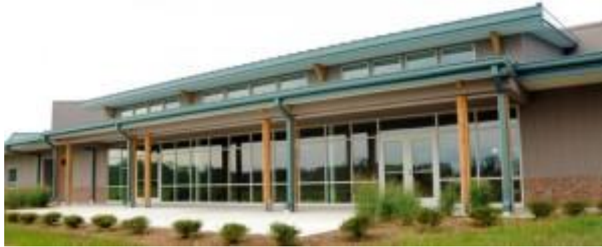
Figure 23: Eastern 4-H Environmental Education and Conference Center in Columbia, NC (Source: sustainability.ncsu.edu)
