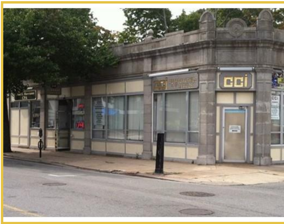
FIGURE 23: VACANT PROPERTY, CABOT STREET, BEVERLY, MA
