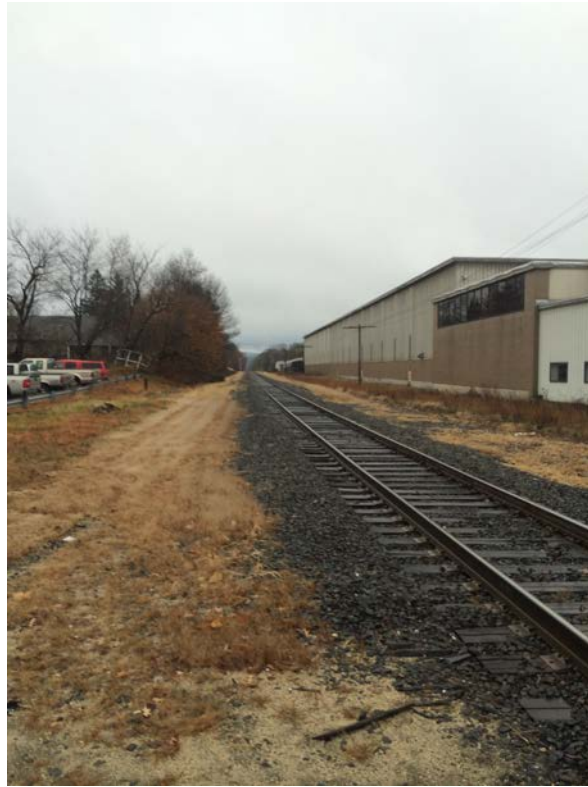
Figure 17: Railway tracks adjacent to Rodney Hunt facility (on right)
