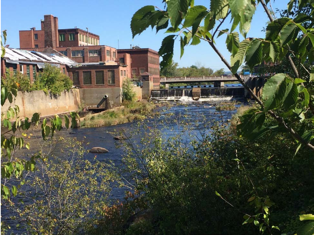
Figure 14: The New Home Sewing Machine Company Dam
