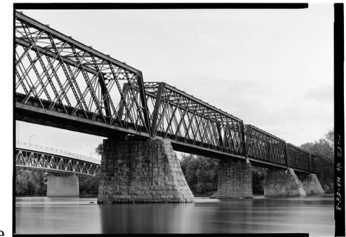
Figure 33: The Northampton Lattice Truss Bridge. Library of Congress
