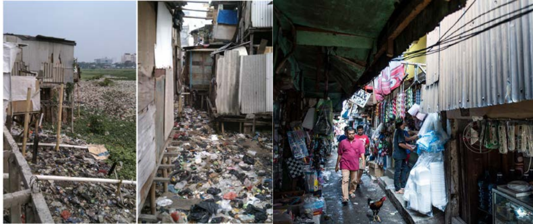
Figure 38: Conditions within Waduk Pluit
