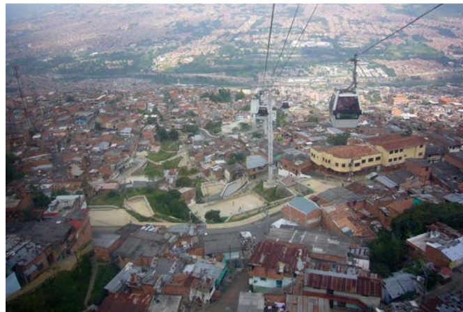
Figure 28: Metrocable serving the PUI
