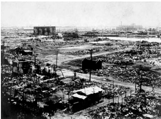
Figure 16: Kanto earthquake aftermath
