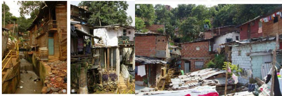
Figure 27: Conditions before PUI project upgrades
