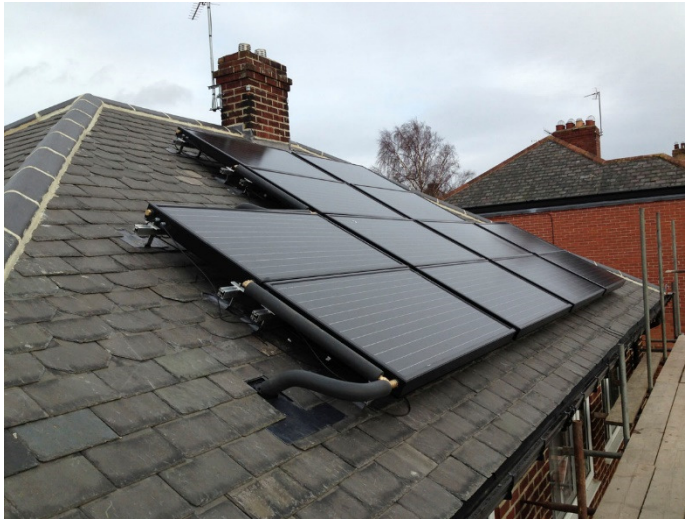
Figure 4. PVT panels come with a more complex installation process due to the need for both electrical and hot water attachments [9].
