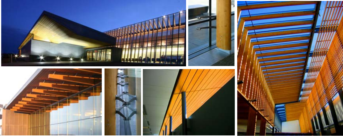
Prince George Airport, British Columbia Photo credit: McFarlane Green Biggar (MBG) Architects
