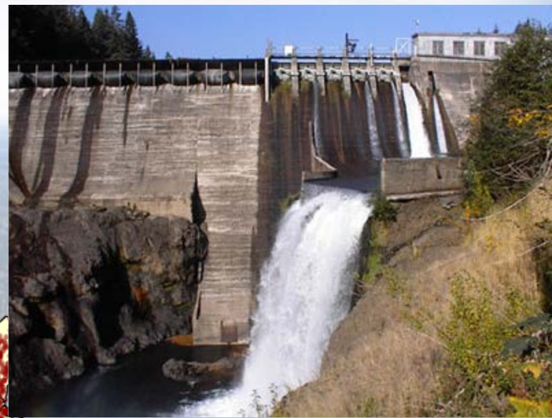
Condit Dam, White Salmon River
