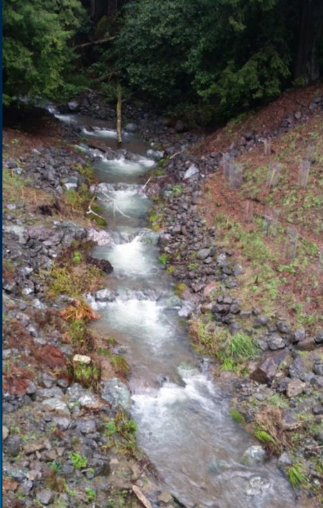
12 Boulder Weirs upstream of Culvert Replacement
