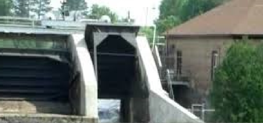
2 Sluice-Tainter Gates 15-ft wide, each end of barrier
