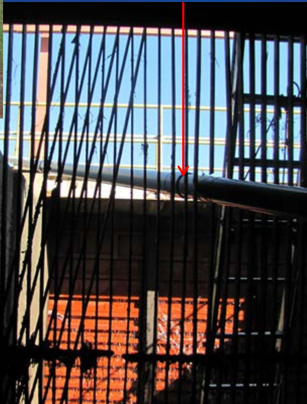
Treatment release pipe going through trash racks
