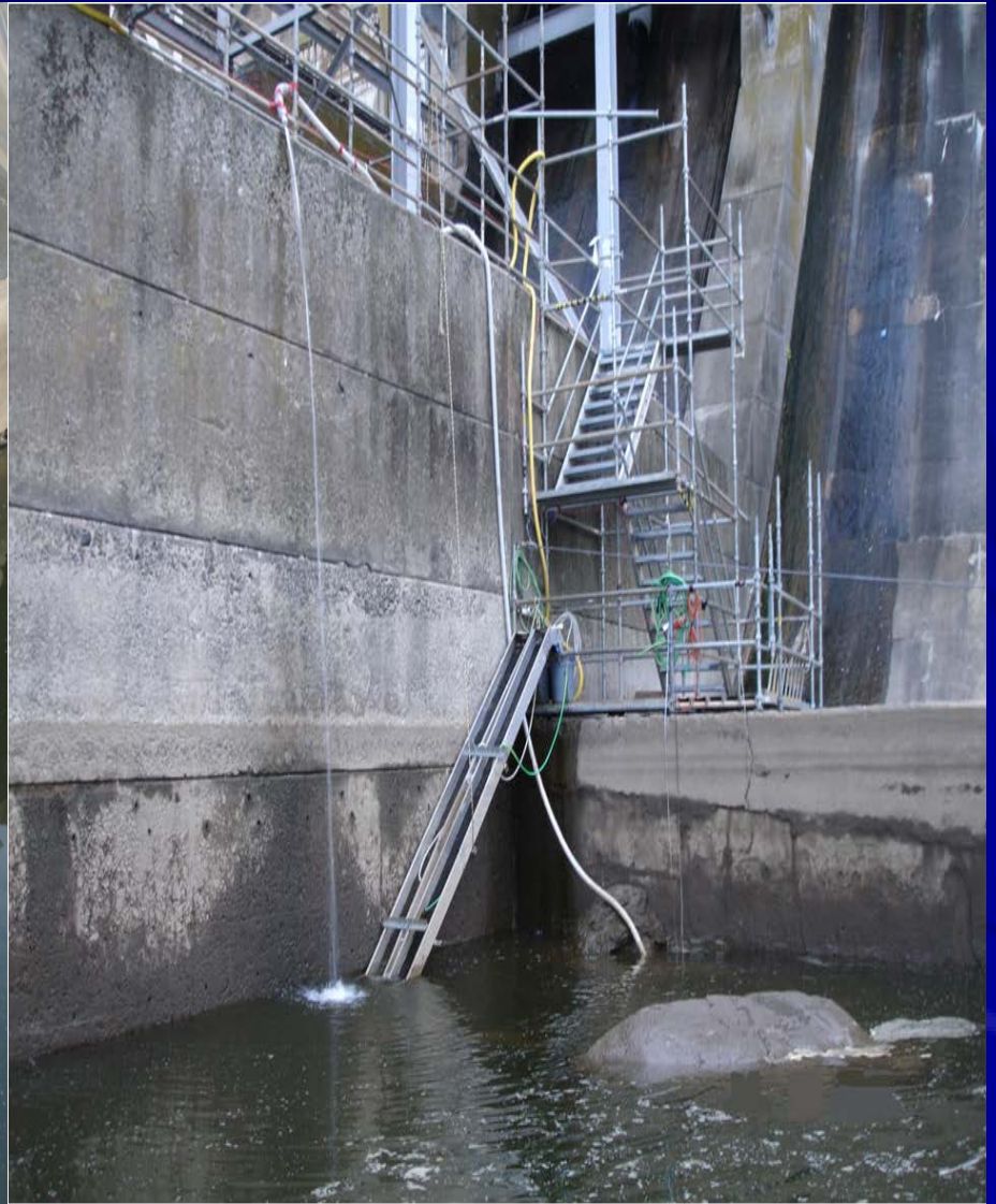
2011 West Ramp Location
