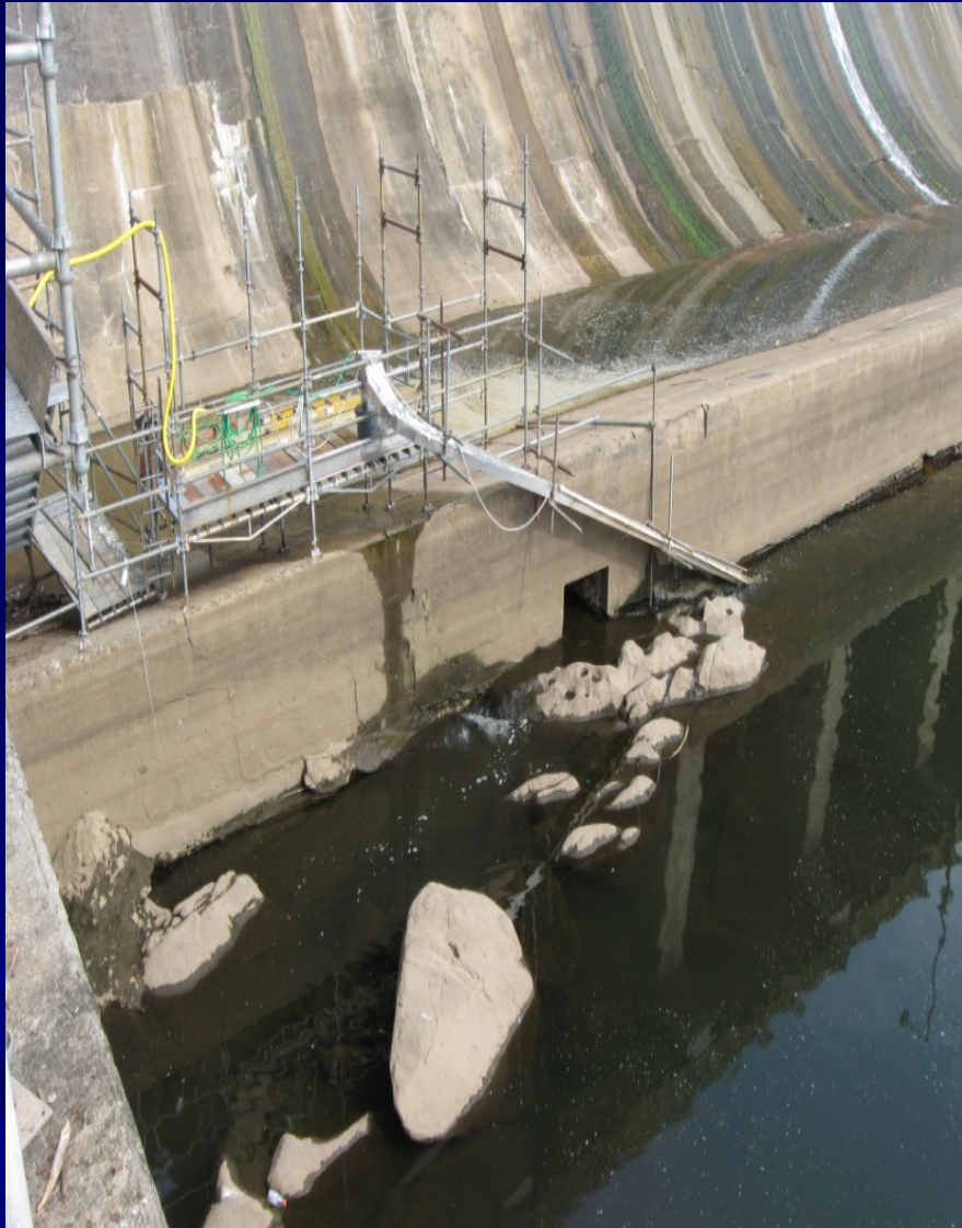
2010 West Ramp Location
