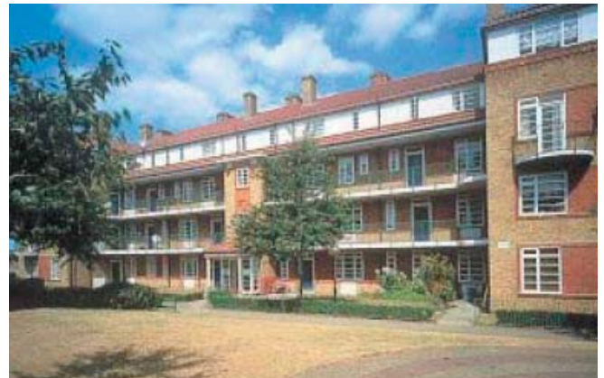
Acorn Walk, Surrey Docks, after refurbishment
