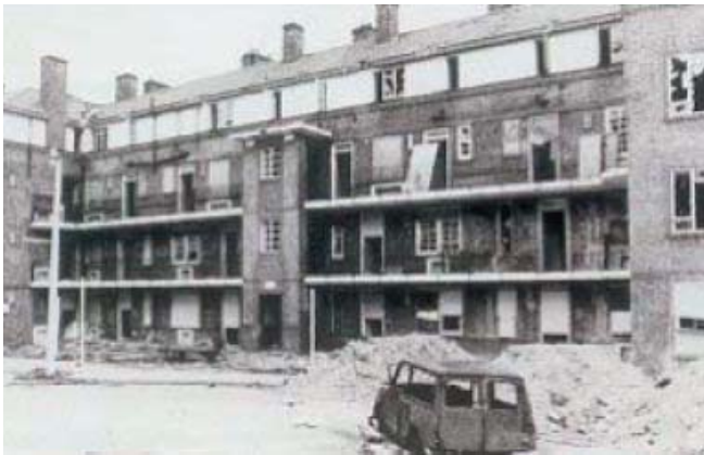
Acorn Walk, Surrey Docks, before refurbishment
