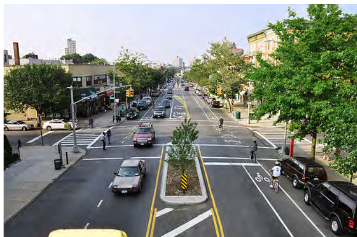
Figure 2.4: Example of how clear, thick, and bright paint, clear signs and lighting can be used to increase safety and wayfinding.
