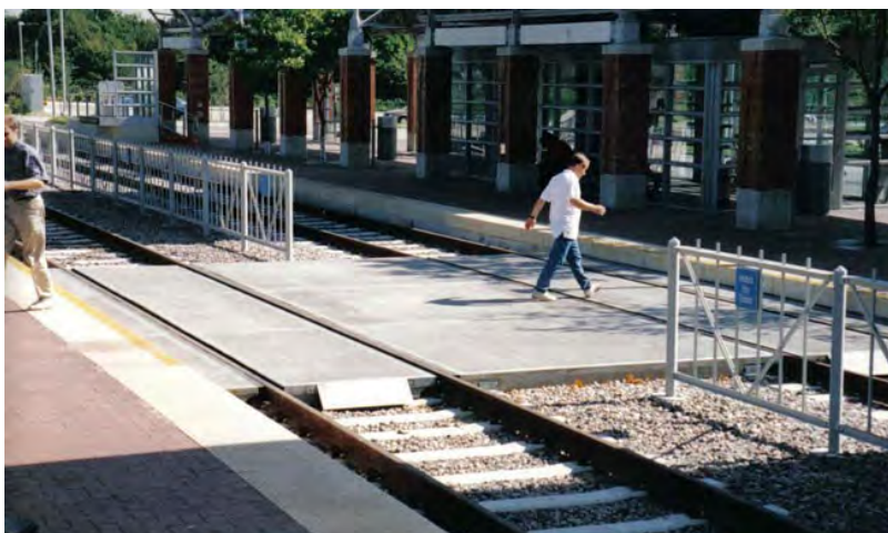
Figure 2.6: A raised crosswalk and gates over railroad tracks helps ensure pedestrian safety.
