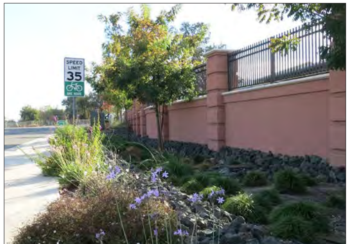
Bioswale already on site at the Derby
