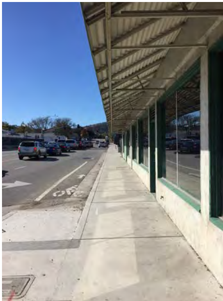
Figure 1.6: Sidewalks along 13th St. have no shade and are falling apart.
