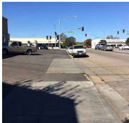
Lot lacks cohesive sidewalks, no barrier between modes, several different cement colors is confusing
