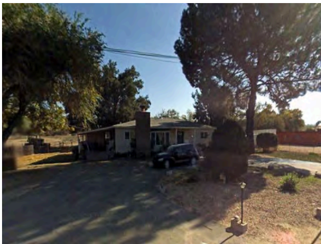
1. View from the left of the residential unit in Lot 12.
