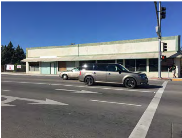
Poorly maintained facade with no landscaping or distinguishing features (vacant lot)
