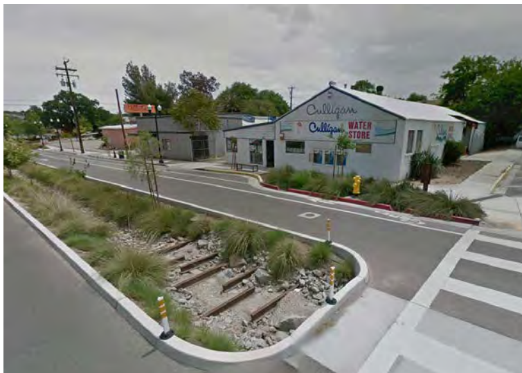
The Paso Robles Street Corridor will include low-impact development bioswales and stormwater management standards such as those in 21st Street to minimize stormwater runoff and pollution into the Salinas River.
