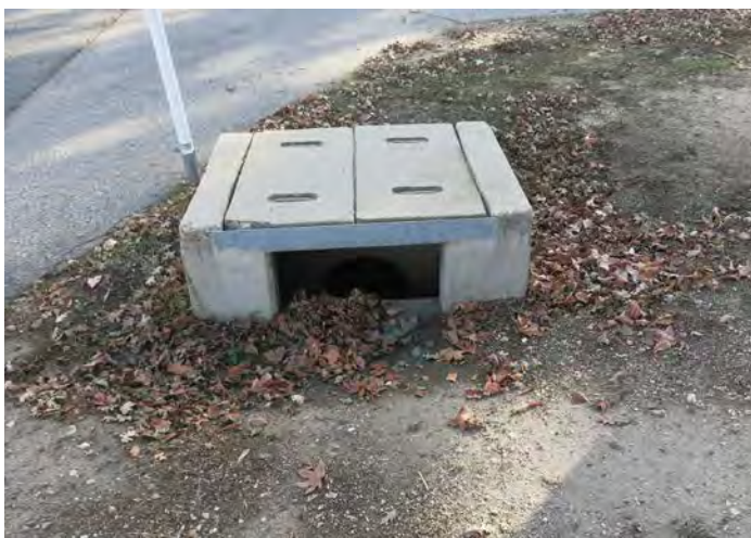
An example existing drainage solution on site
