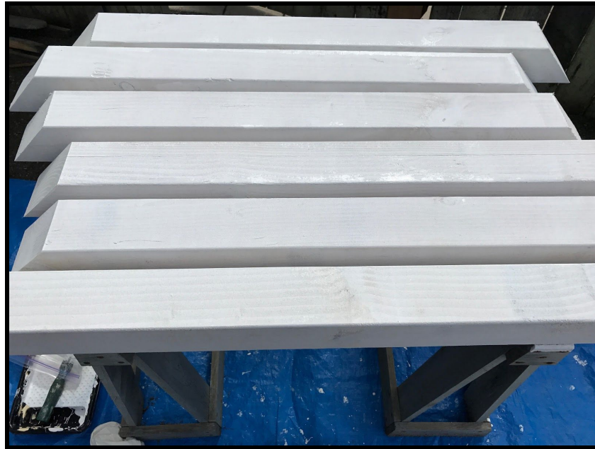
Figure 65. An image of the struts being painted.
