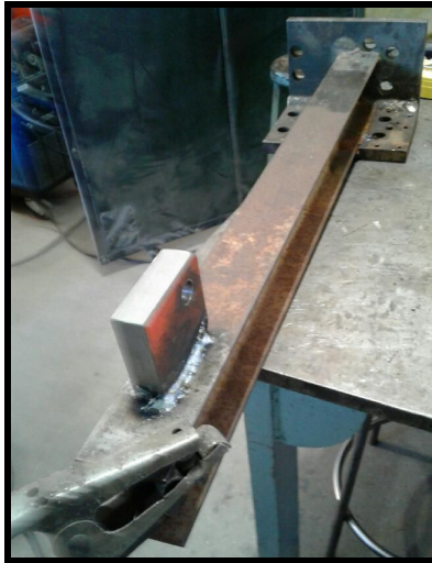
Figure 52. An image of the attachment plate after it was welded to the pre-welded structure.
