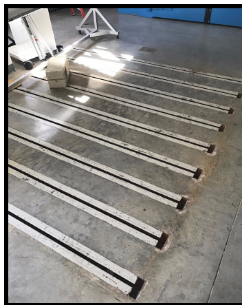
Figure 1. An image of the strong floor in the Composites Lab that our steel scaled model and testing fixture will bolt into.
