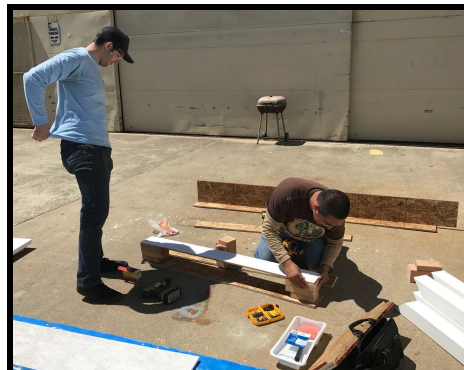
Figure 63. An image of Austin and Octavio assembling the column assembly.
