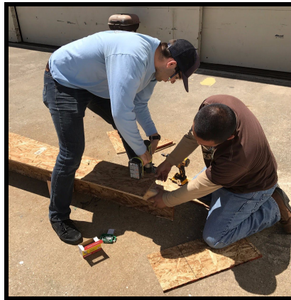
Figure 62. An image of Austin and Octavio assembling the beam assembly.
