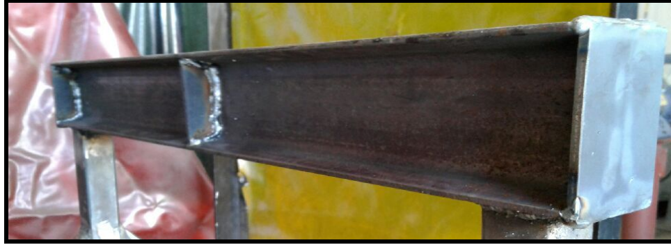
Figure 50. An image of the I-beam after the end plates and gussets were welded on.
