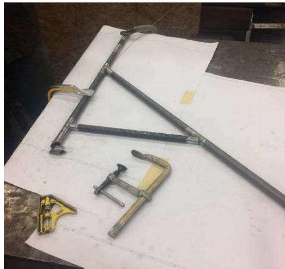
Figure 5.1.2 One side of the frame being fixtured against a 1:1 printout before being tacked together.
